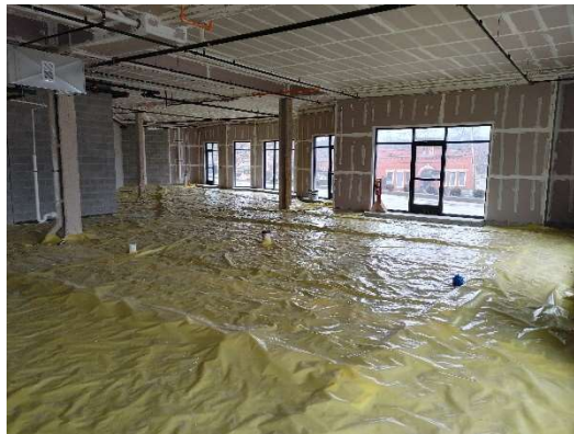
Interior Space, looking SE
