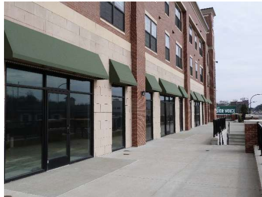
Side Plaza on East Market St.
